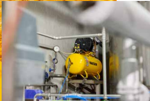
The Friedmann brewery has relied on compressed air from KAESER reciprocating compressors for many years.
