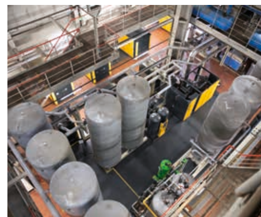
Two different compressed air treatment systems dry the compressed air for the respective requirements.
