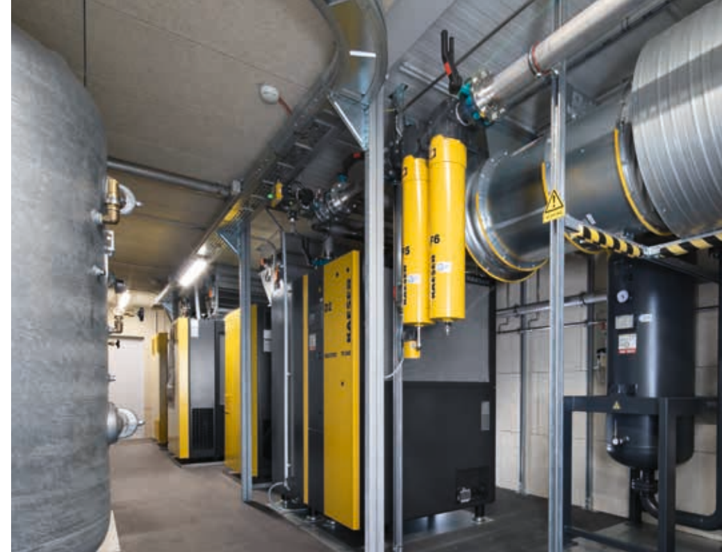
The container housing the compressed air station has been completely lined with sound insulation mats to comply with sound emission limits.
