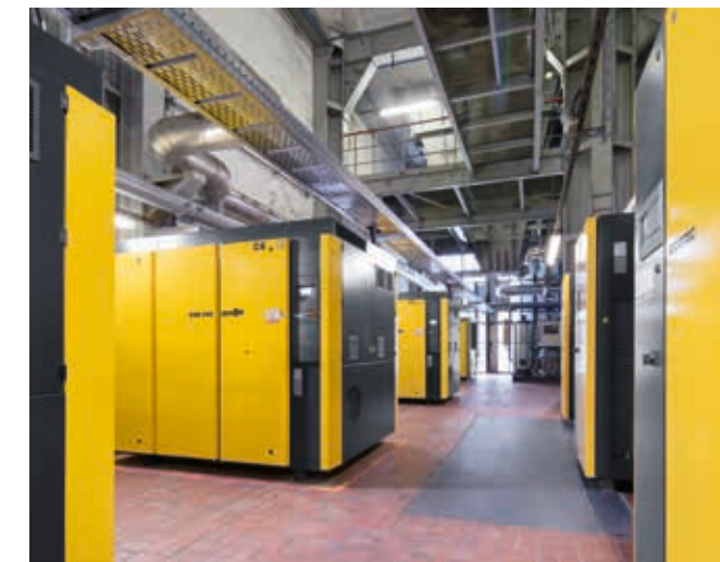
A total of four rotary screw compressors with IE4 drive motors and the energy-saving SIGMA PROFILE operate in the compressed air station.
