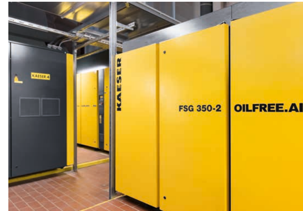
Compressed air fulfils a number of important functions at the Hanover facility, including transportation of the lead oxide.
