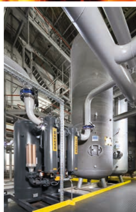
The 70,000-litre storage volume is divided between eight compressed air receivers.
