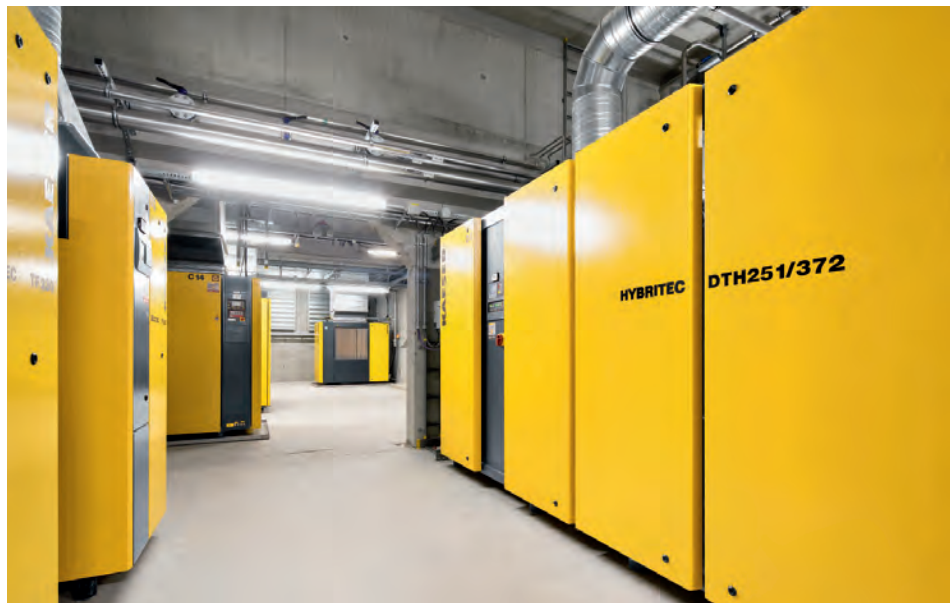
The new compressed air station, which includes a HYBRITEC combination dryer.
