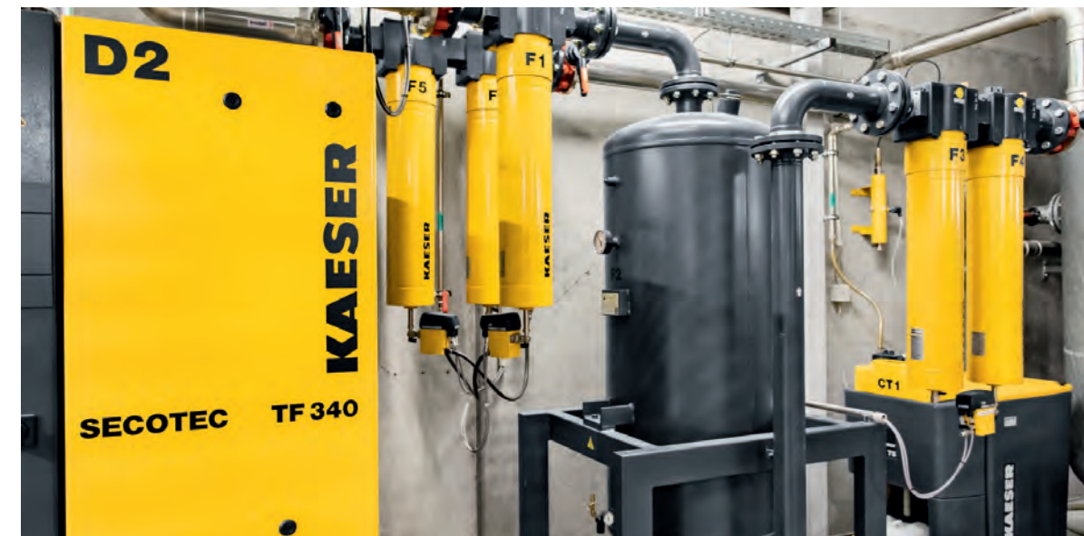
To ensure that the compressed air supply meets the required purity and quality standards, the system includes two TF 340 refrigeration dryers, as well as activated carbon adsorbers and a variety of KAESER filters with remarkably low pressure losses.
