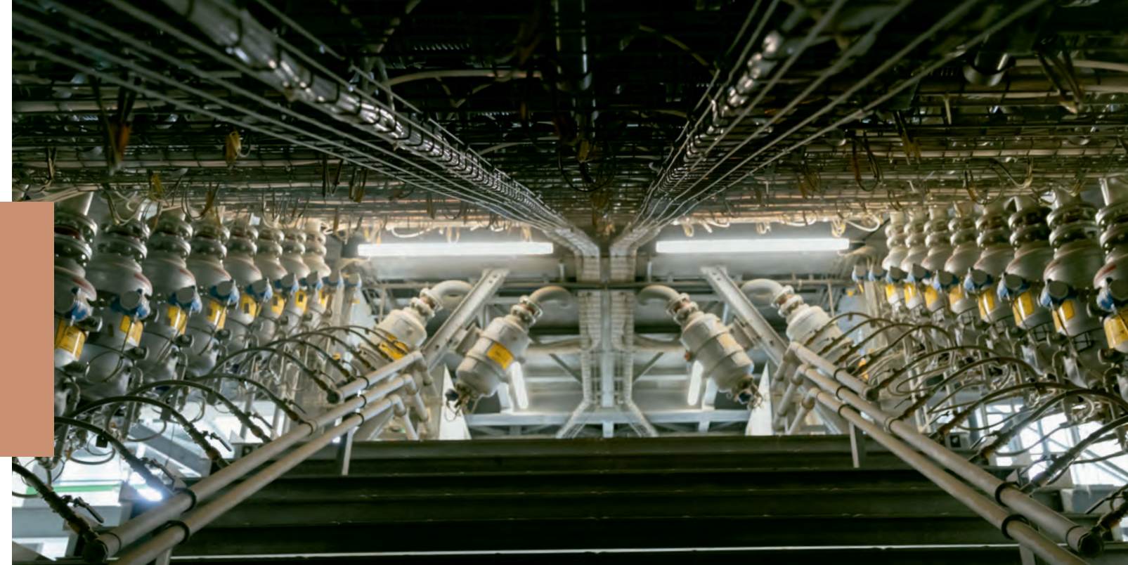
Compressed air distribution below the combustion chamber.
