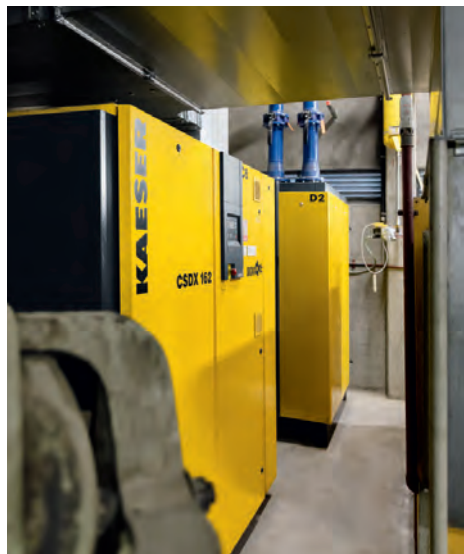
Part of the old compressed air system. It distributes compressed air subject to stringent dryness requirements.
