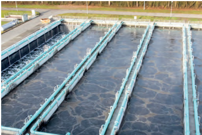
Compressed air is used to supply oxygen for the microorganisms active in the clarification tanks.
