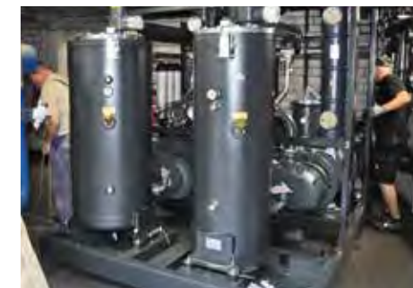
The rotary screw compressor system made a long and arduous journey: first, it was dismantled and lowered through the light shaft into the lower level of the building.
