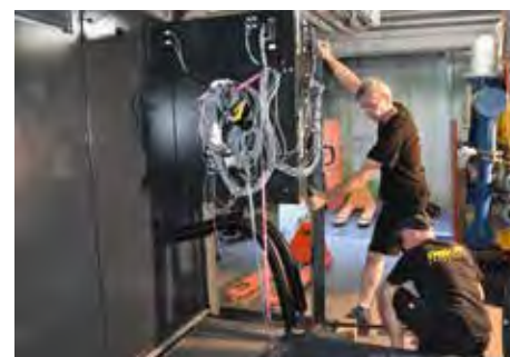
The rotary screw compressor system made a long and arduous journey: first, it was dismantled and lowered through the light shaft into the lower level of the building.
