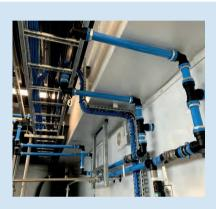
As the sole Scottish Registered Distributor for **EQOfluids UK** pipe systems, Kerr Compressors has vast experience of designing and installing reliable pipework systems to provide efficient distribution of compressed air, nitrogen, vacuum and oil around customer factories, manufacturing facilities or specialist zoned areas and applications. A unique and versatile product range, the EQO range is colour coded to comply with the type of media being transported.
